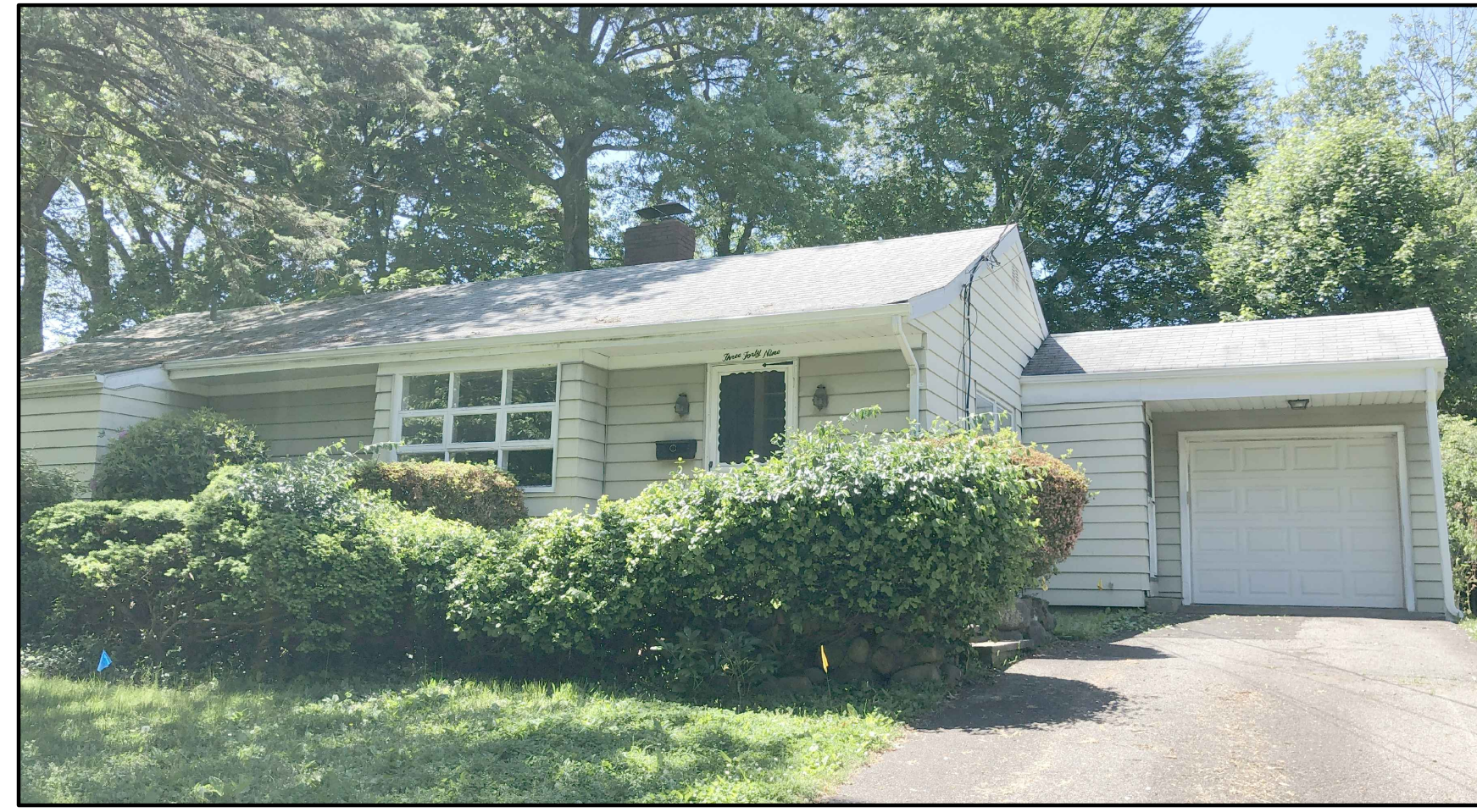
EXISTING CONDITIONS PHOTO
