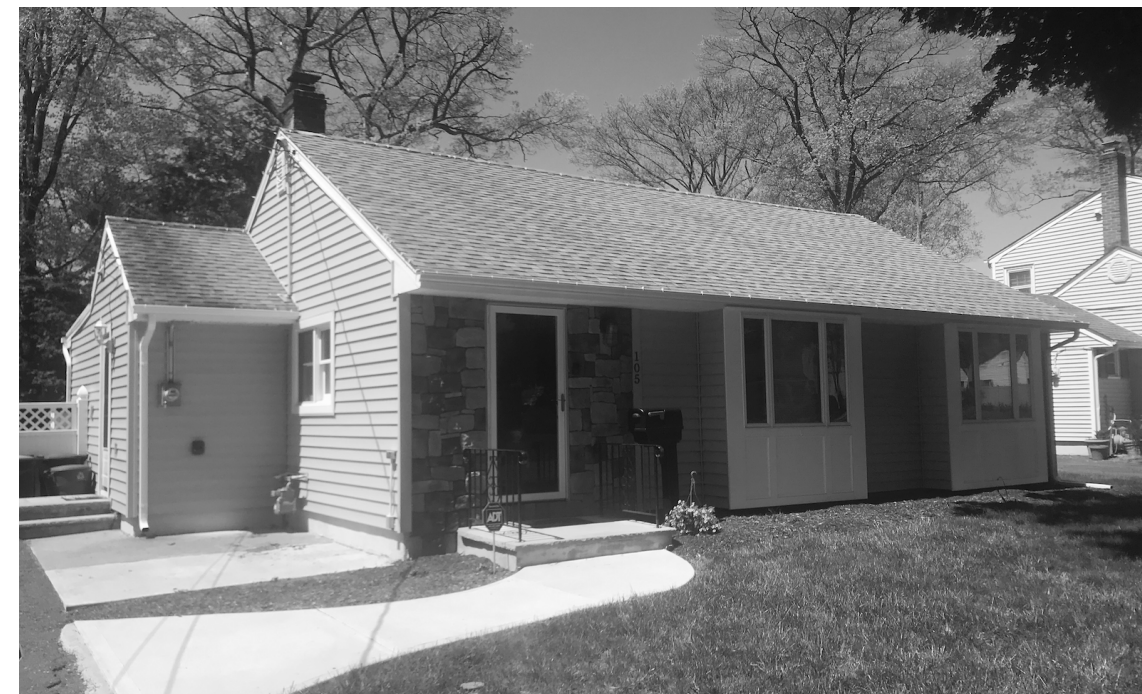
VIEW OF EXISTING BUILDING
