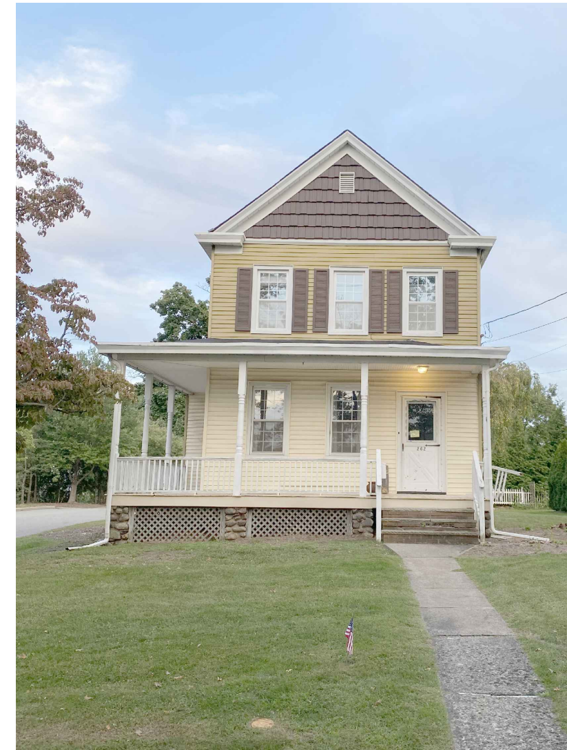
EXISTING CONDITIONS PHOTO
