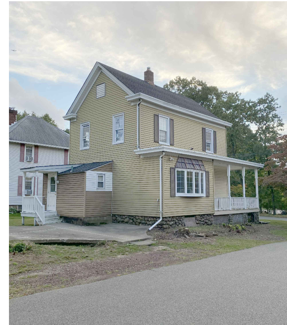
EXISTING CONDITIONS PHOTO
