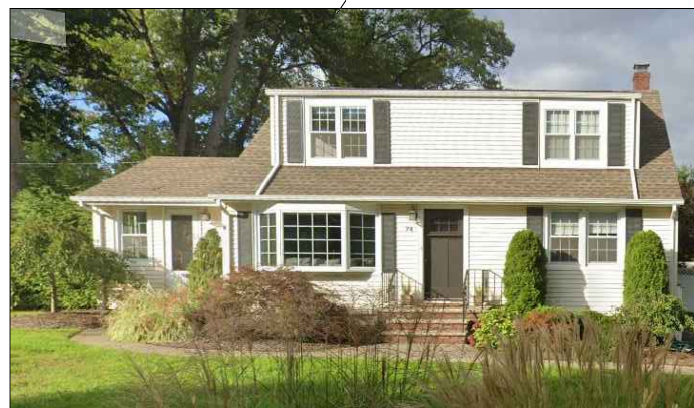
EXISTING BLDG. PHOTO (FRONT)
