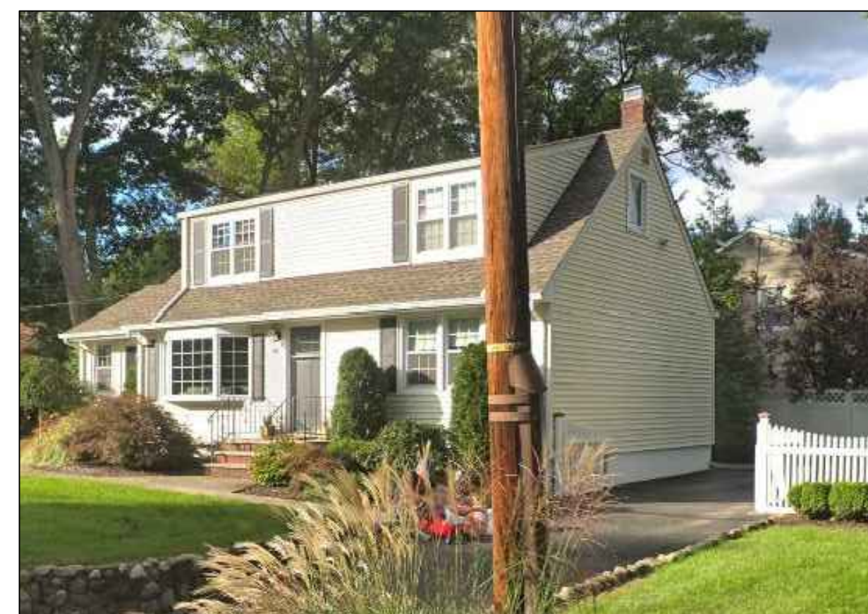
EXISTING BLDG. PHOTO (RIGHT SIDE)
