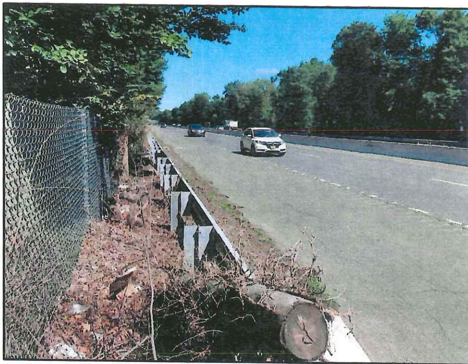
Photograph 10: View to the northwest of proposed culvert replacement along Route 208 SB
