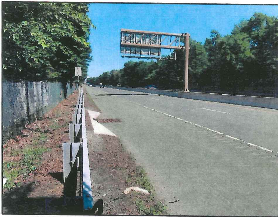
Photograph 9: View to the northwest of proposed guiderail replacement along Route 208 SB
