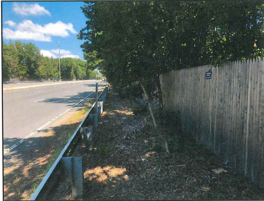
Photograph 7: View to the northwest of the fence running adjacent to Route 208 NB
