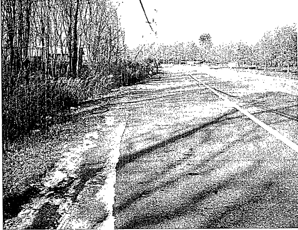
Photo 5: Typical location of a gas distribution main in the left shoulder of the roadway, adjacent to wetlands
