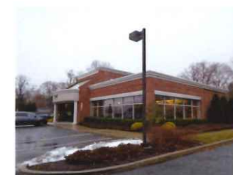
PHOTO 2 (SIDE BUILDING VIEW)
